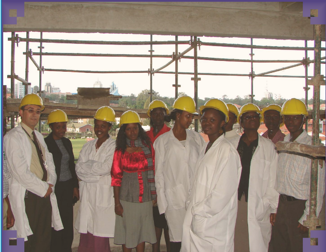
Students taking a tour of the Students Centre building under construction
